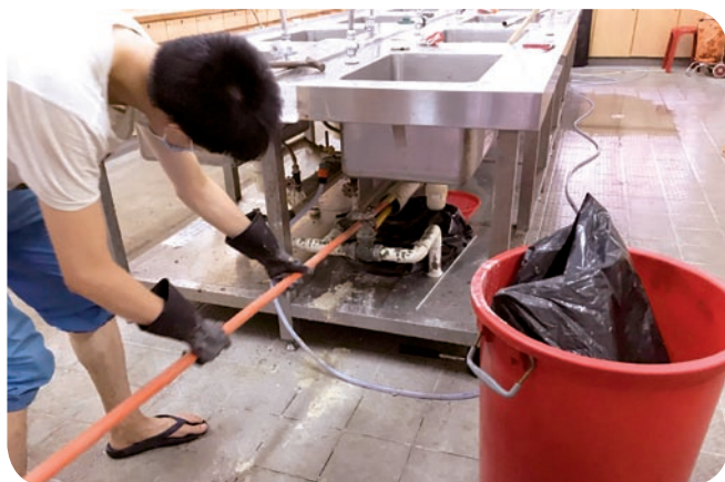
高華閣舍友義工協助宿舍清理淤塞喉管 Lodger of High Street House assisted to clean up blocked pipes
